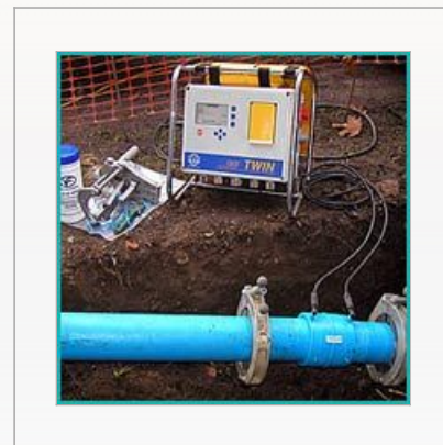
Electrofusion Welding
